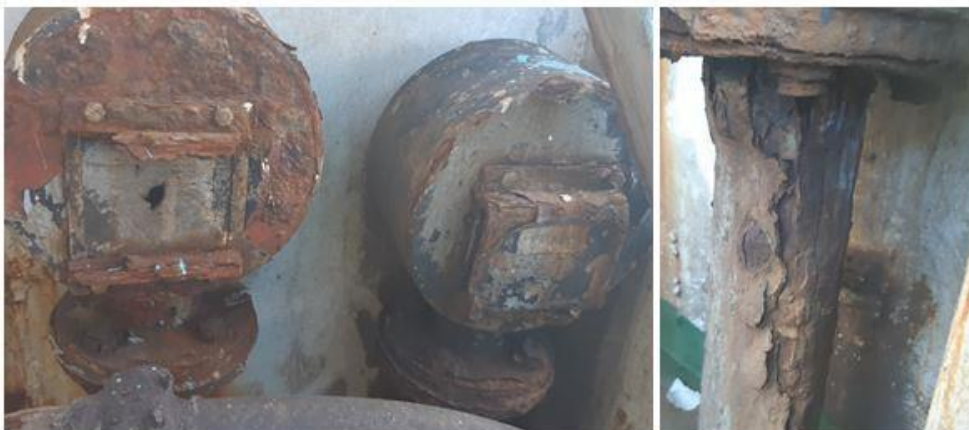
Figure 3 Heavy corrosion on starboard side fuel vents in area of gangway.
