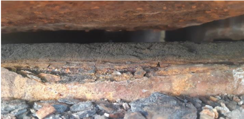
Figure 18 Cargo hatch does not seat correctly on the compression bar (port side).
