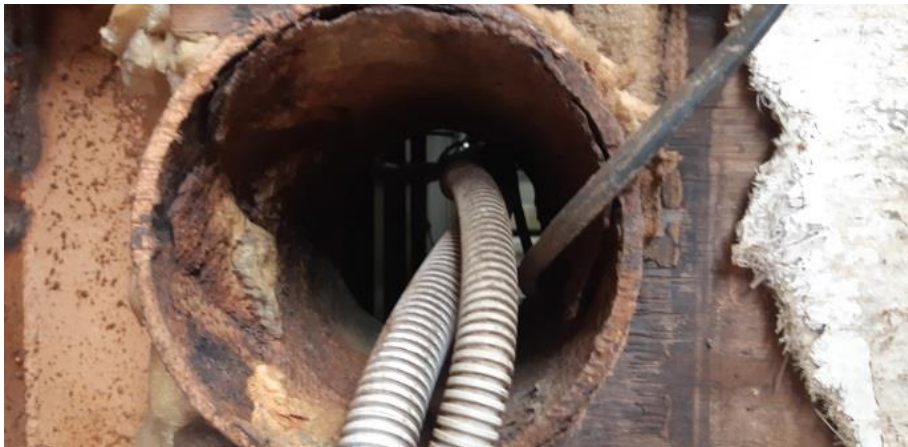
Figure 24 View into engine room from cargo space.
