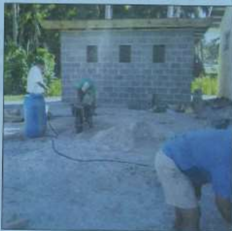
Workers constructing sanitation facility in Mitiaro.
