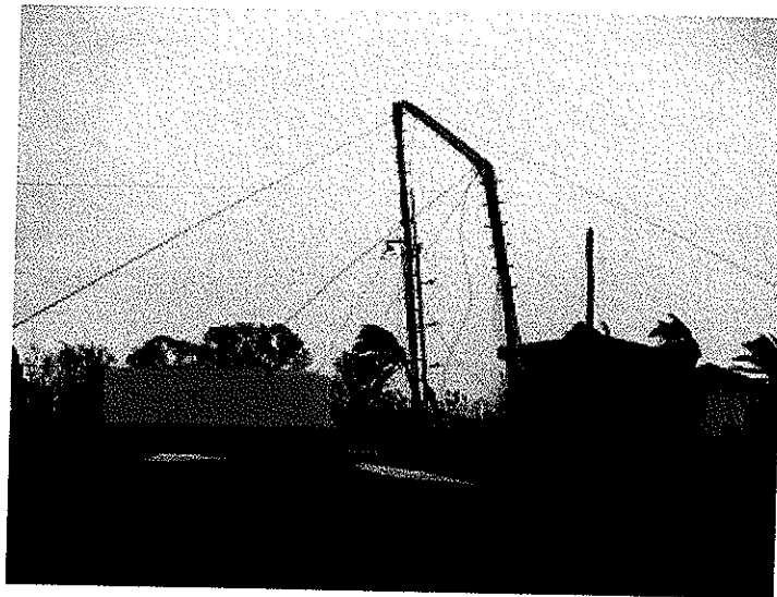
Damaged Telecom mast in Aitutaki after it was damaged by TC PAT in the early hours of the morning of February 10 th , 2010
